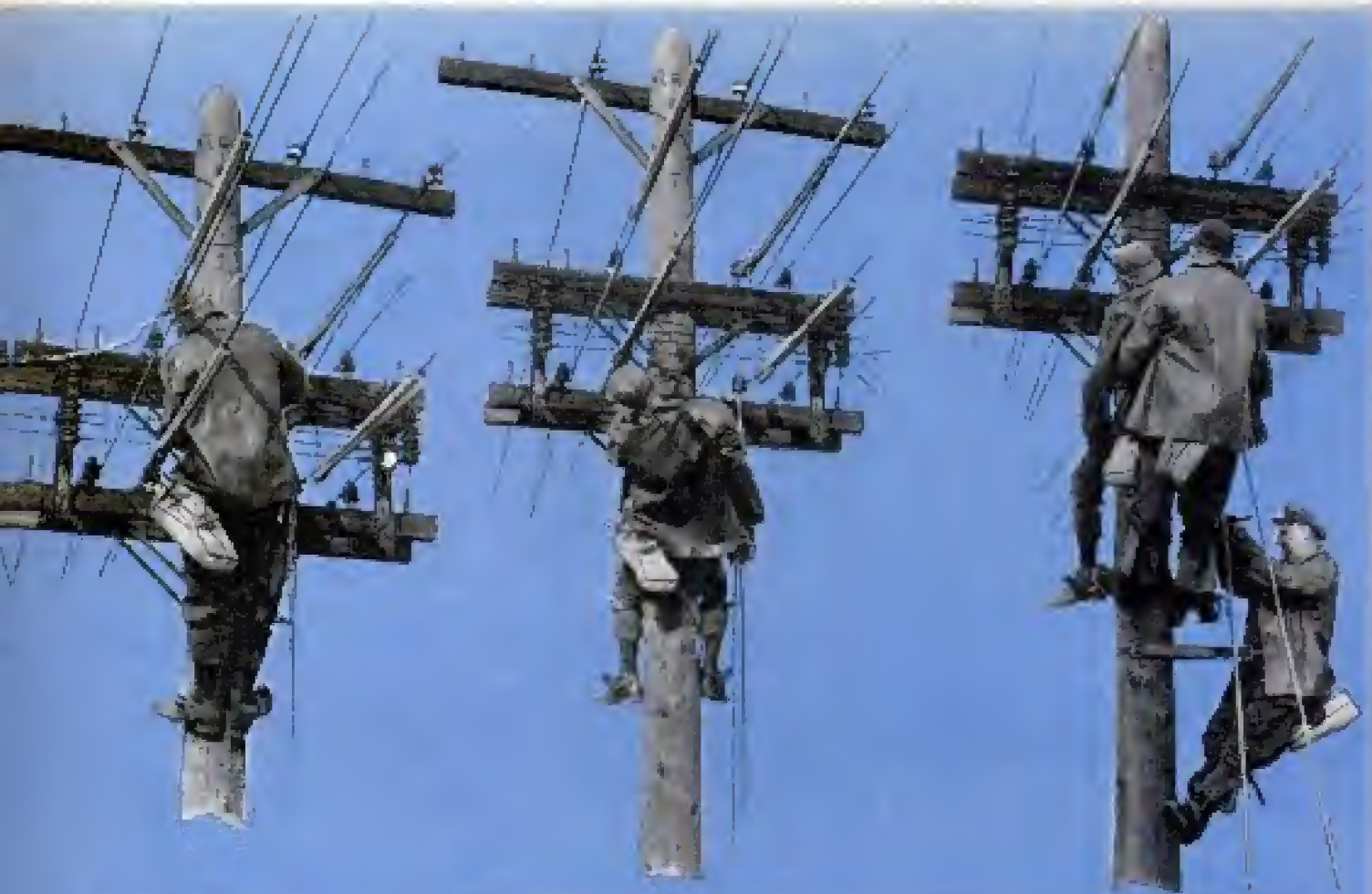
Trouble men of Philadelphia Electric carry out a mock pole-top rescue. Rubber guards placed over line have slipped back, exposing "hot" wire. Worker brushes his head against wire and is knocked unconscious. He falls back against his safety belt and fellow workers rush up pole. One unfastens the victim's safety belt while the other throws a line under his arms and over the crossarm on the pole. Victim is gently lowered to the ground and co-workers administer artificial respiration.
